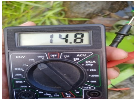
Figure 5. Generator Voltage Measurement for 1 Minute
