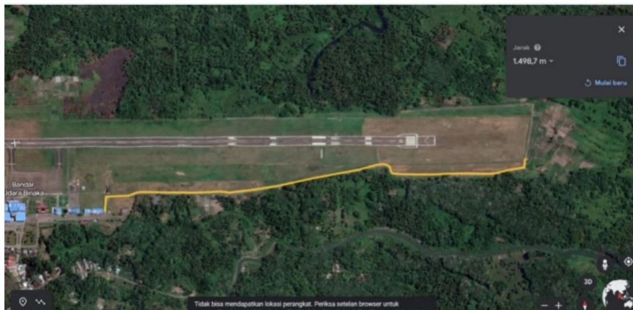
Picture 3: Inspection Road Perimeter Runway 27 Binaka Airport Gunungsitoli
