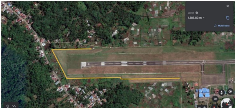
Picture 4: Inspection Road Perimeter Runway 09 Binaka Airport Gunungsitoli
